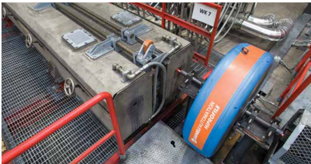
HiPROFILE LITE plant installation
