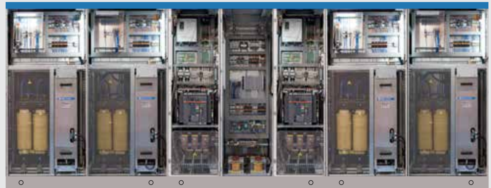
INVERTER UNIT #1 | INVERTER UNIT #2 | INCOMING LINE #1 | CONTROL SECTION | INCOMING LINE #2 | INVERTER UNIT #3 | INVERTER UNIT #4
